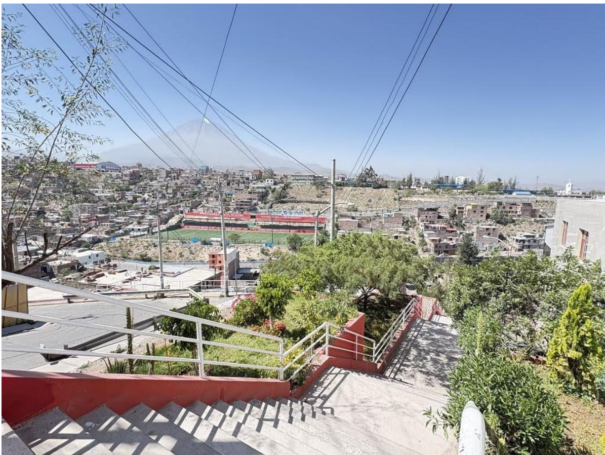
Figure 3. Municipal intervention in Cayma, Arequipa. | Photo. The authors
